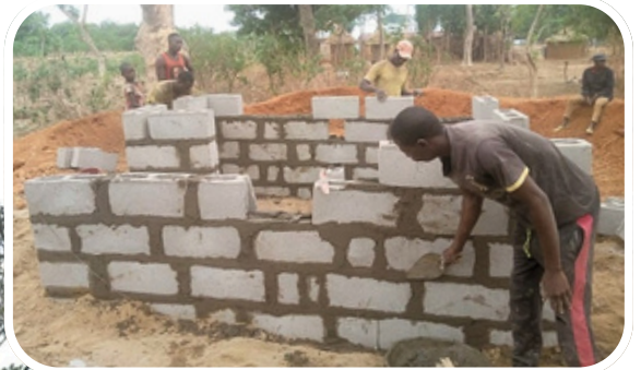
Puluko community latrine construction
