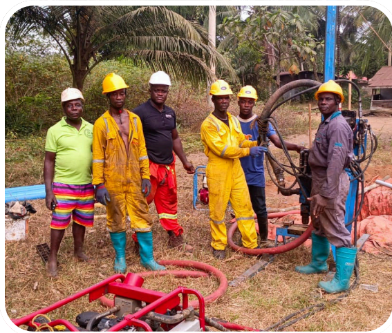
The team drilling the first well in River Cess County
