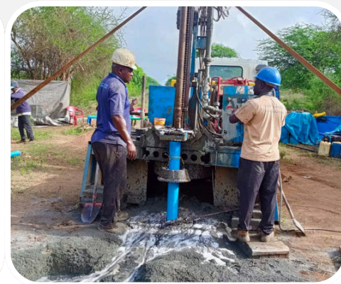
Drilling a new well in Kwa Muthui, Kenya
